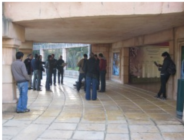
Fig. 2.14. Large slabs set in concrete with deep grouting
