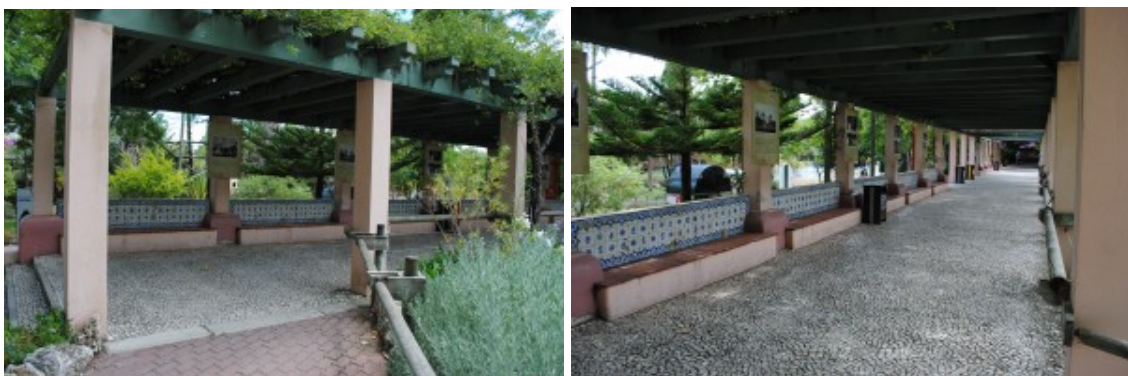
Fig. 2.20. Left: transition from interlocking brick paving, over concrete bands, to Portuguese pavement. Right: a long stretch of Portuguese pavement under a pergola
