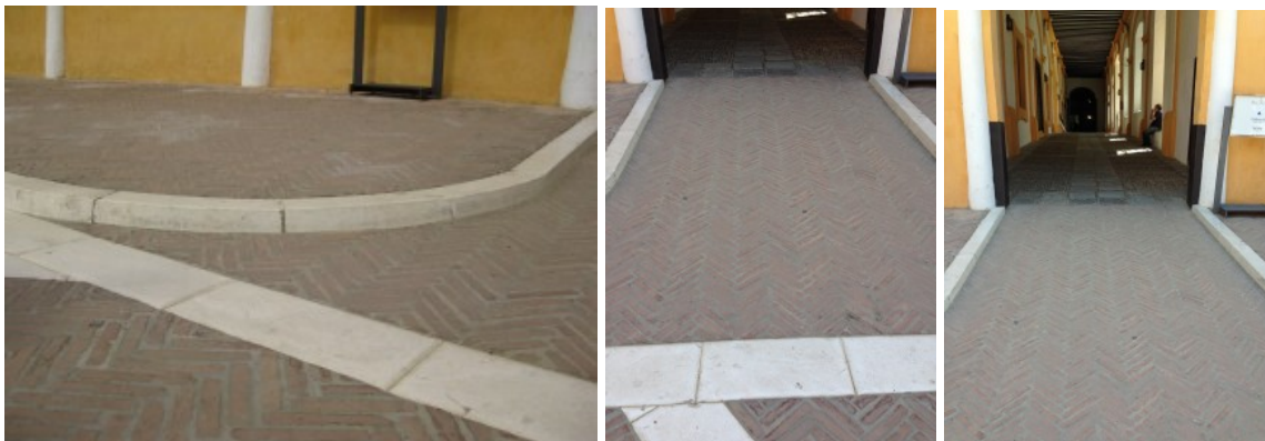
Fig. 2.6. Left: one of the curbs before the covered walkway. Middle and right: slightly inclined transition from fields of rougher dark red bricks herringbone laid in concrete between smooth white stone slab dividing lines to fields of cobblestones laid in concrete between flagstone slabs.
