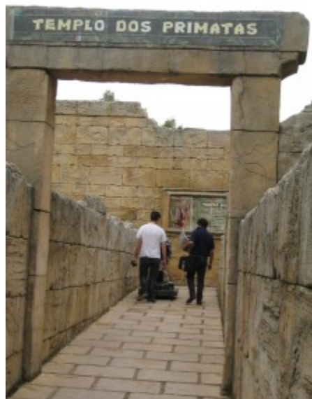
Fig. 2.22. Large stone slabs laid in concrete with wide grouting and a hairpin bend at the top of the incline Once inside the Temple, the surface is smooth concrete painted red (Figure 2.23).
