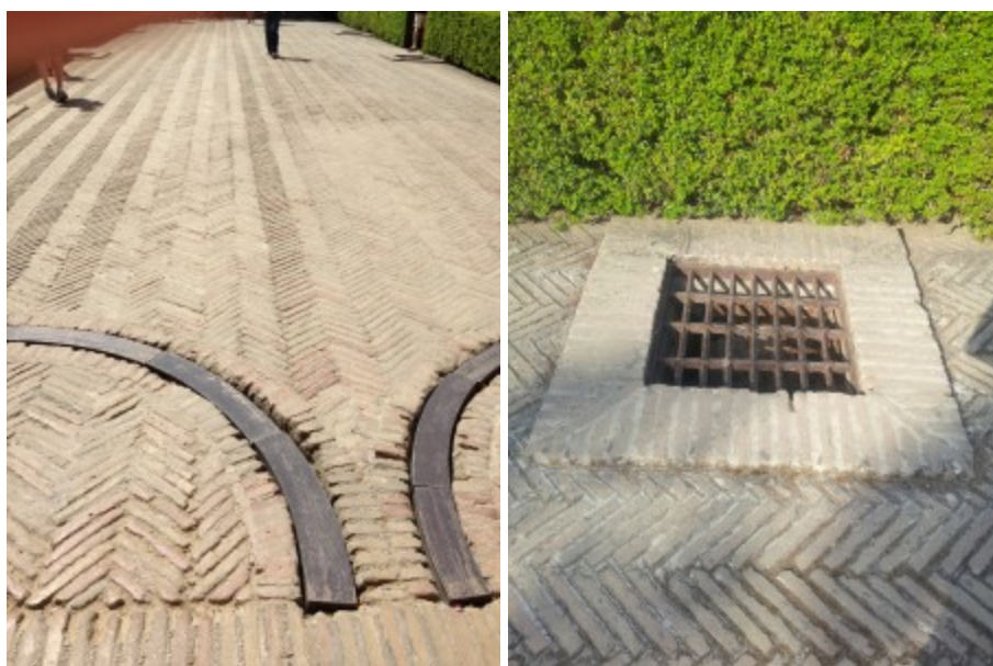
Fig. 2.8. Left: overview of herringbone laid brick Crossing Court showing gate wheel gutters with wooden fillers. Right: air vent grate in raised brick surround along herringbone laid brick path.
